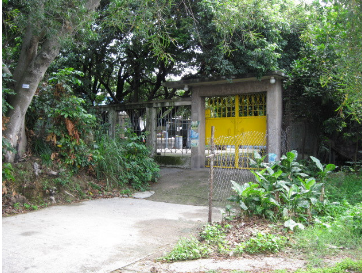
▪ Photo 64 N19 Village House
