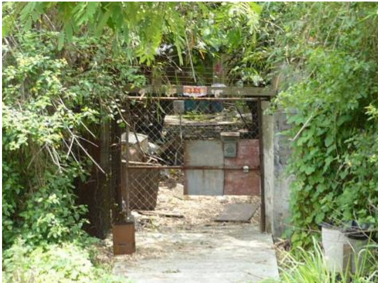
▪ Photo 68 N23 Village House
