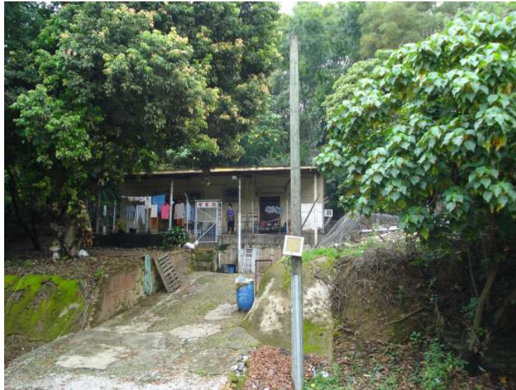
▪ Photo 67 N22 Village House
