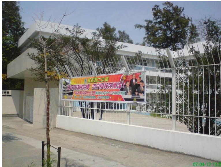
Photo 55 N13a (Fung Kai No. 1 Secondary School, No.1 & 2 Primary School & Kindergarten)
