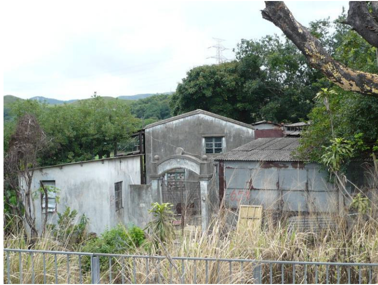
▪ Photo 69 N24 Village House
