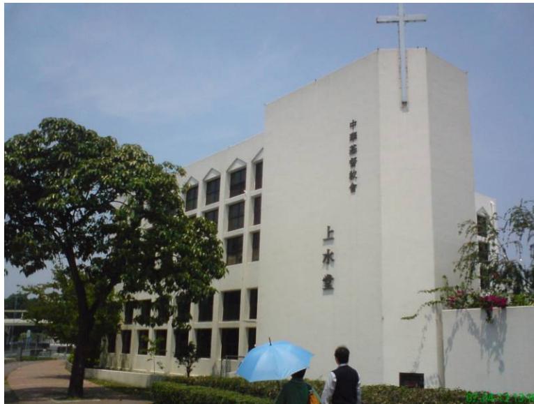
▪ Photo -59 N14 (Sheung Shui Church)
