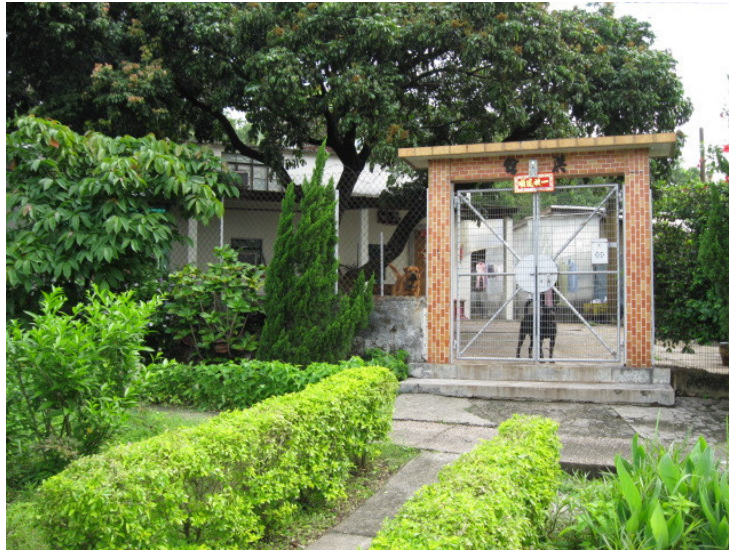
▪ Photo 63 N18 Village House
