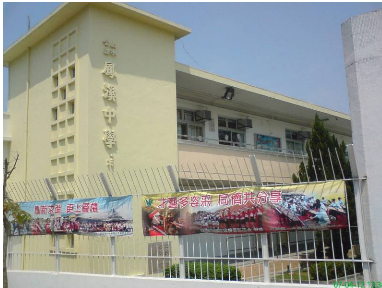
Photo 56 N13b (Fung Kai No. 1 Secondary School, No.1 & 2 Primary School & Kindergarten)
